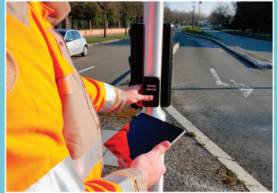
“Getting started with the controller” Commissioning and maintenance of equipment at distance (1m away from the material and up to 80m from the controller)
